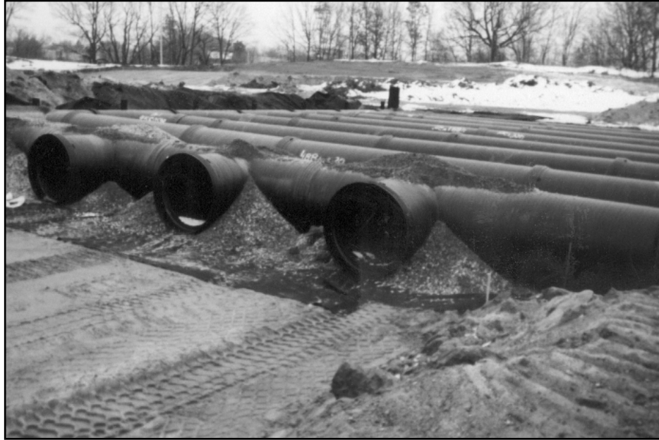
Figure 3-5: On-Site Storm Water Detention Facilities
